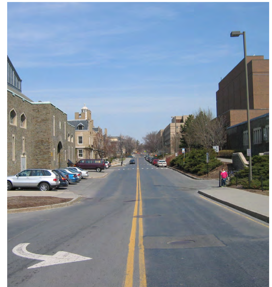
Garden Avenue, existing conditions, looking north from Campus Road
