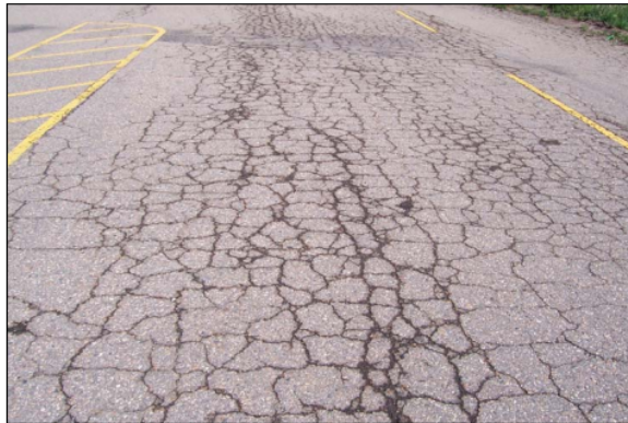
FIGURE 4: High Severity Alligator Cracking
