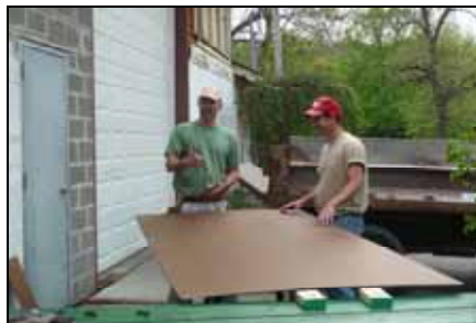
Volunteers replacing broken windows with wood to be painted as trompe l'oeil windows.
