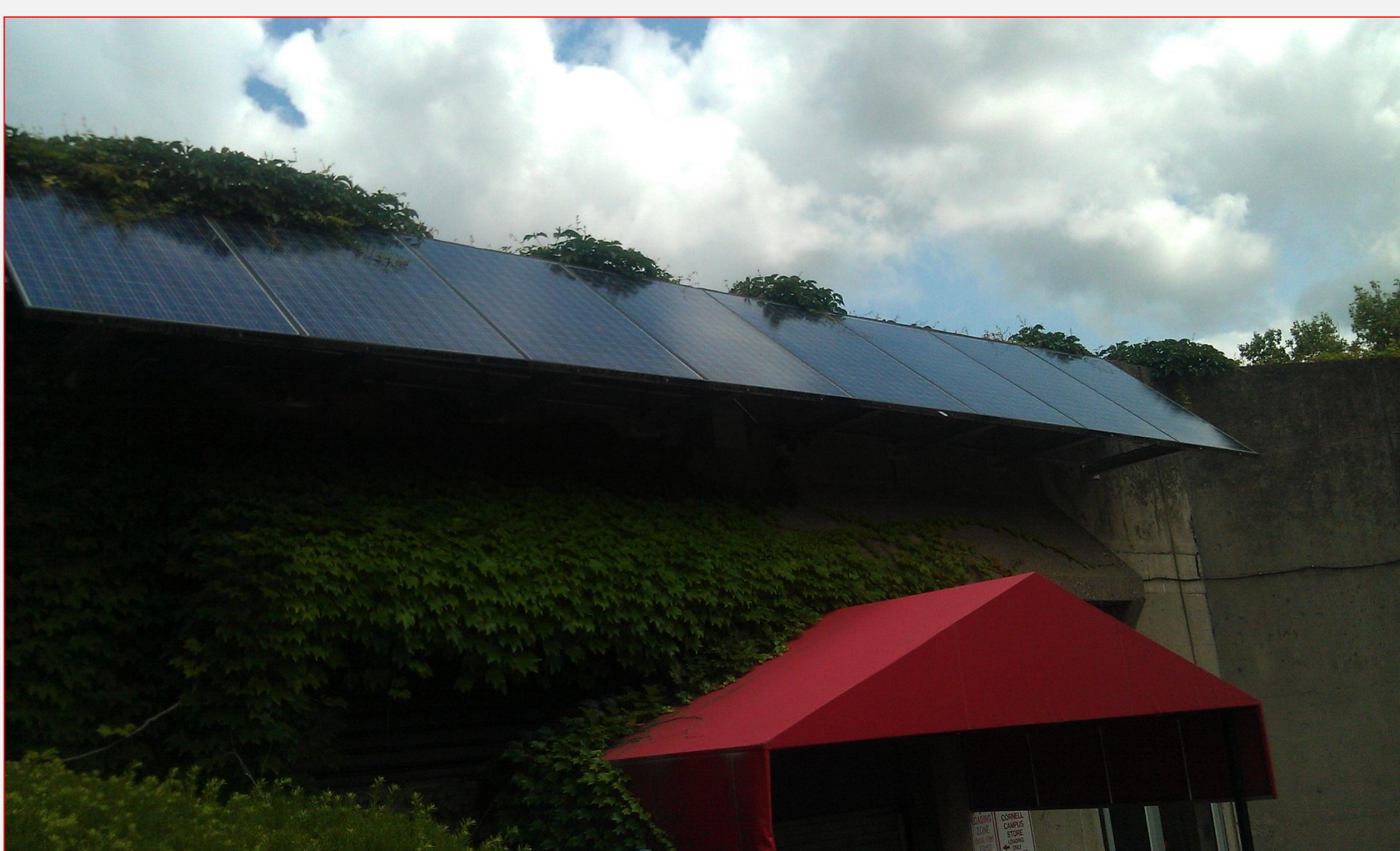
The Cornell Store 2.2 kilowatt system
