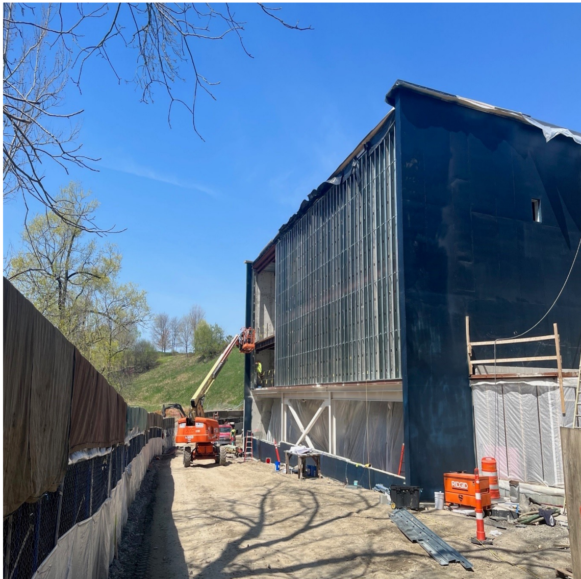
Metal Framing Installation Along South Wall of NEH High Bay
