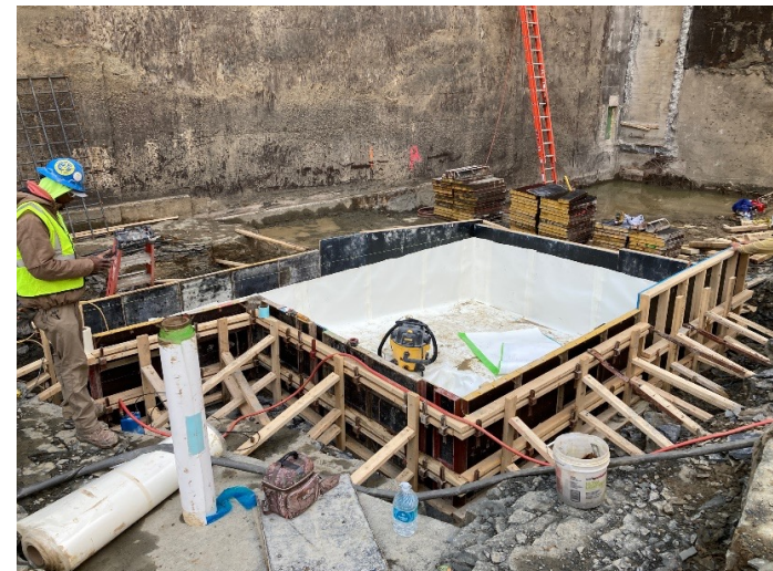
Waterproofing elevator pit
