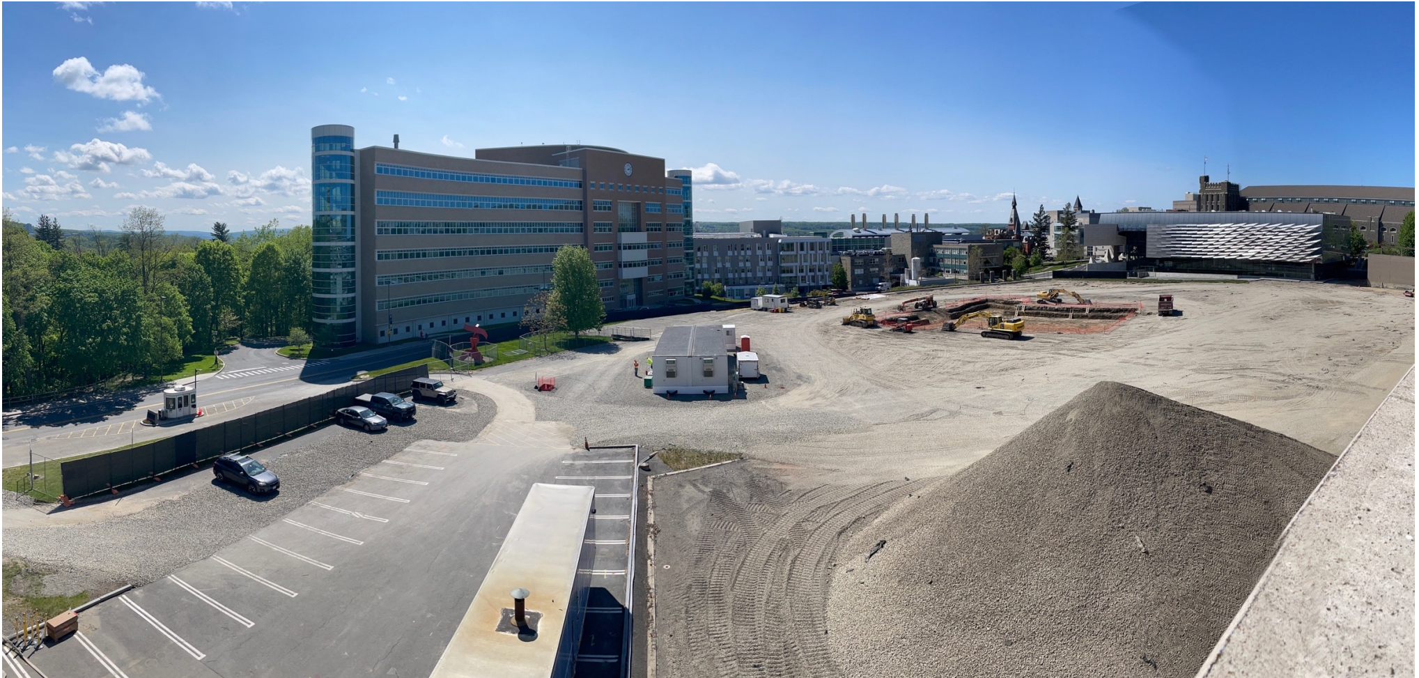
Sitework in Progress
