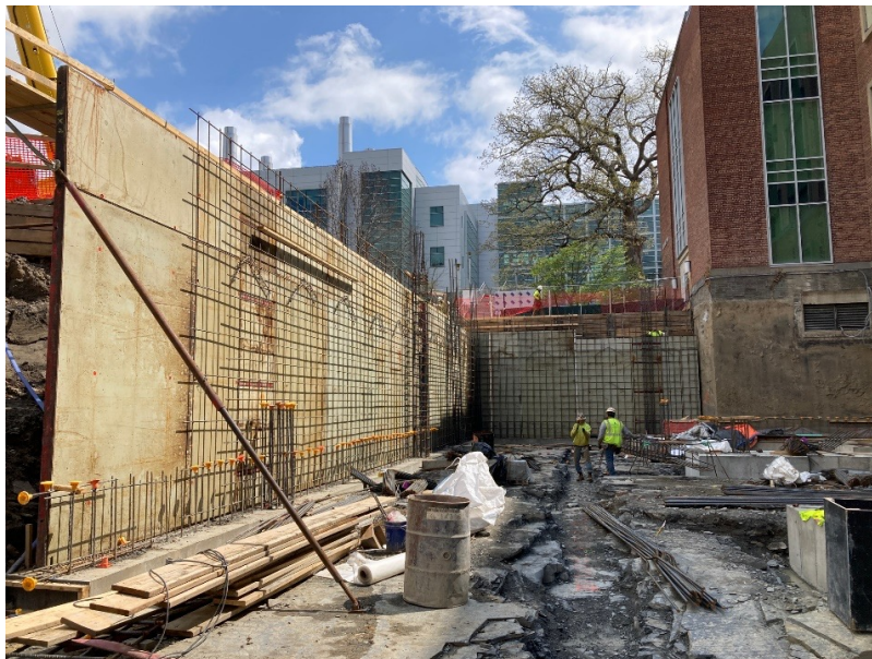
Foundation walls rebar and formwork
