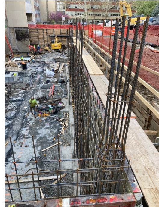
Foundation walls rebar and formwork
