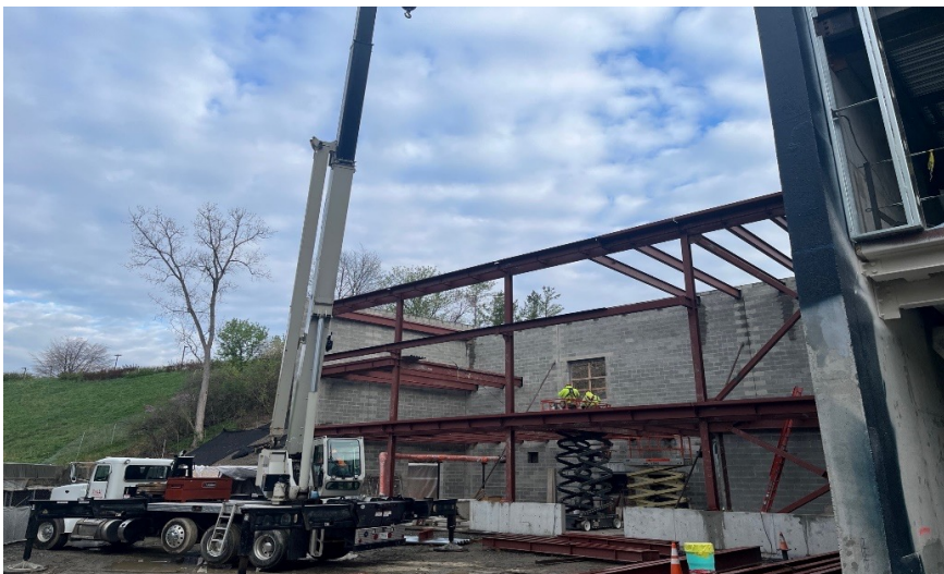
Steel Erection Ongoing at Sector Seven
