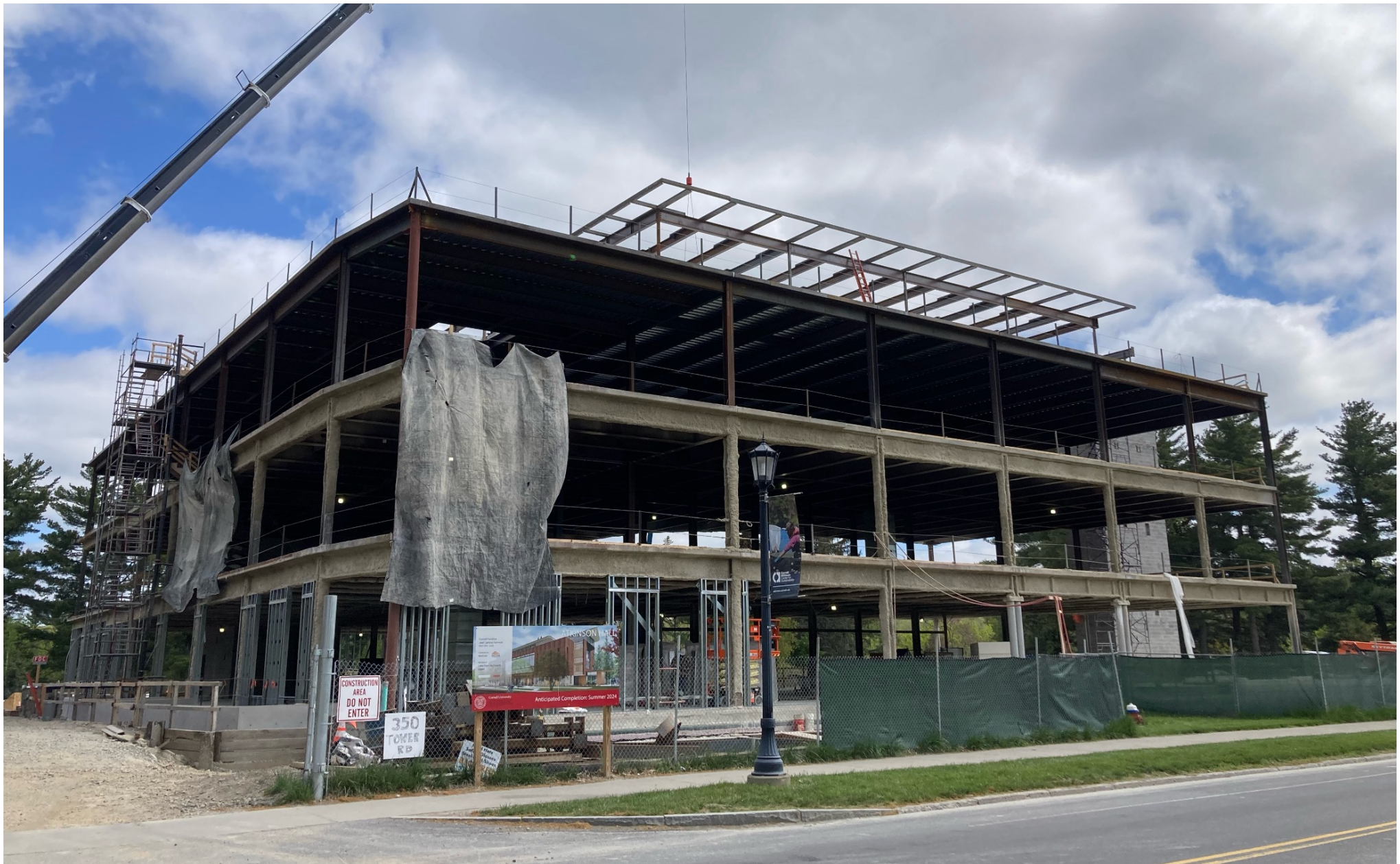
Structural steel frame
