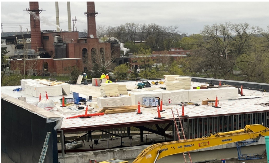
High Bay Roof Placement Underway
